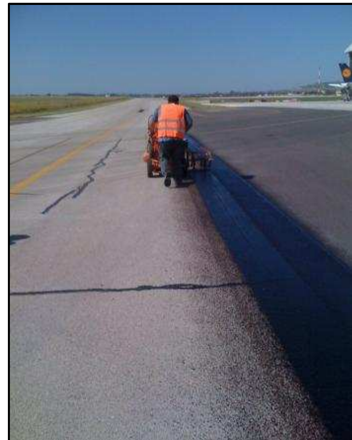
Rhinophalt application on the Taxiway Lima surface
