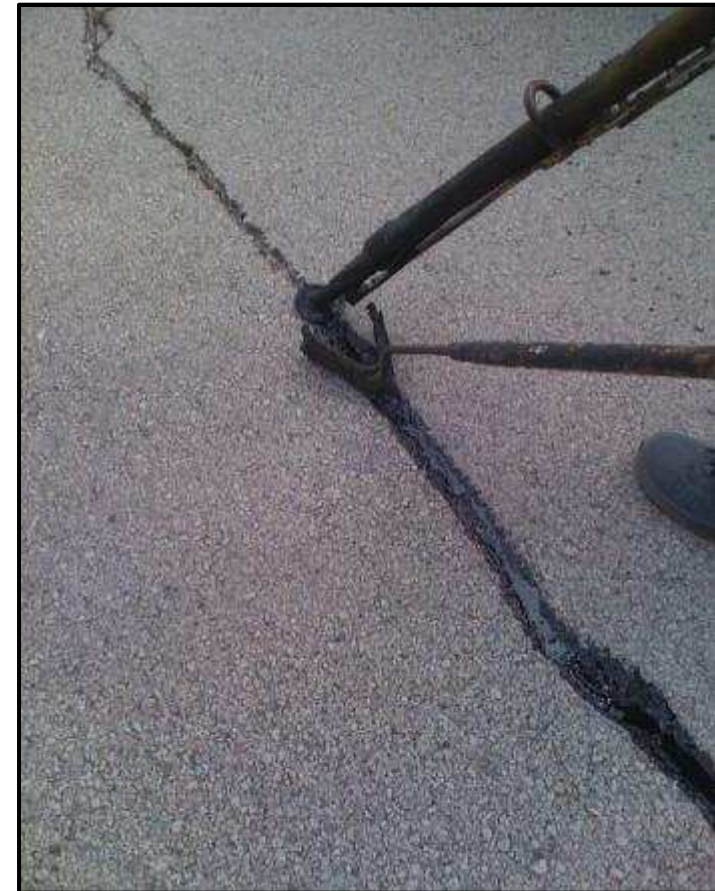
Cracks Sealing on M.I.A. asphalt pavement
