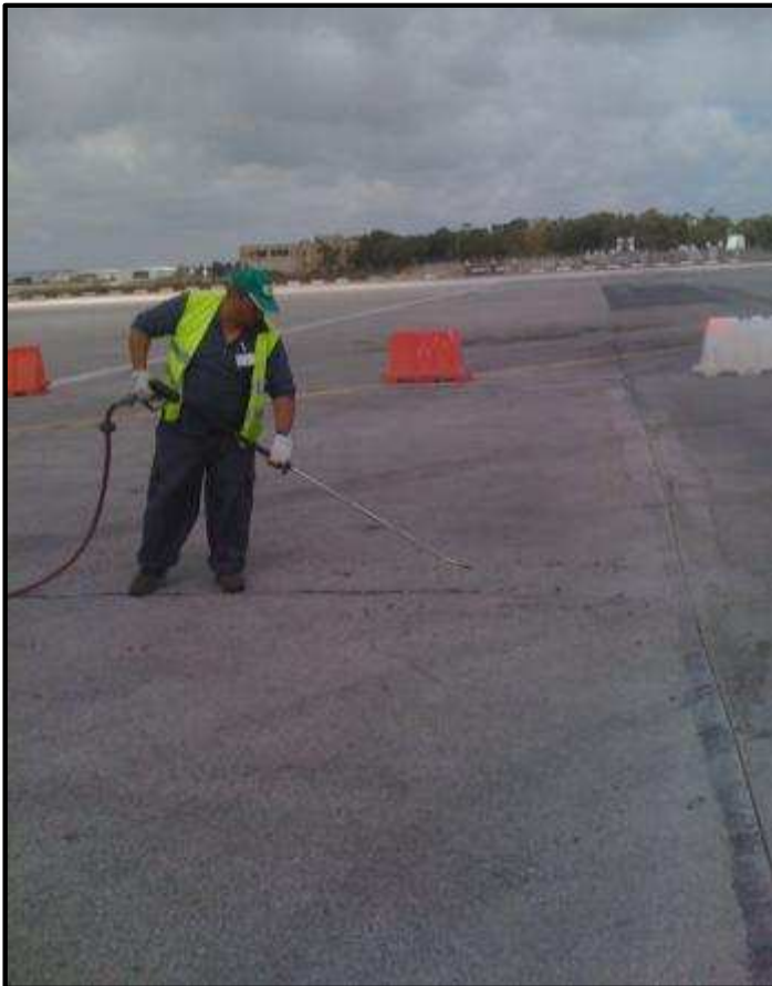
Cracks cleaning
